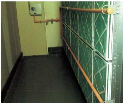
*The VESDA by Xtralis air-sampling pipe network does not interfere with the fan filters or ongoing maintenance at the Wells Fargo Center in Minneapolis.*
