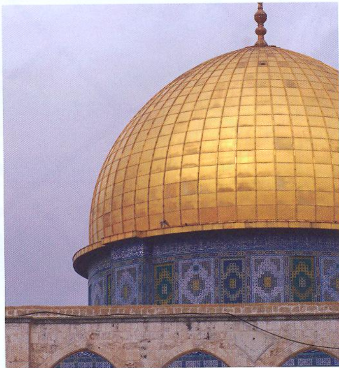
■ The Xtralis system will help protect the Dome of the Rock from damage by fire.
