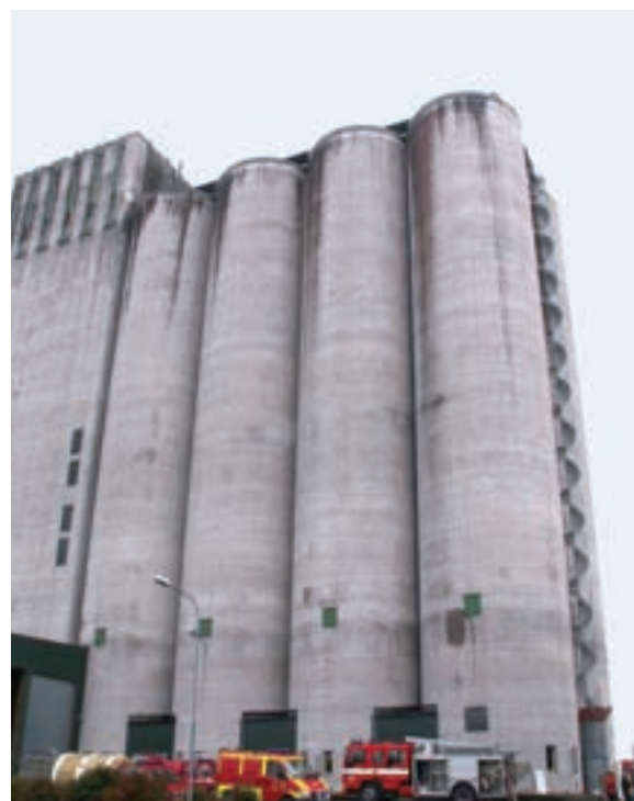
Figure 5: the silo on fire (second from right) was 47m high, 8 m in diameter, and filled to about 40m with wood pellets. A vaporisation unit was used to ensure that the gas was injected in gaseous phase.
