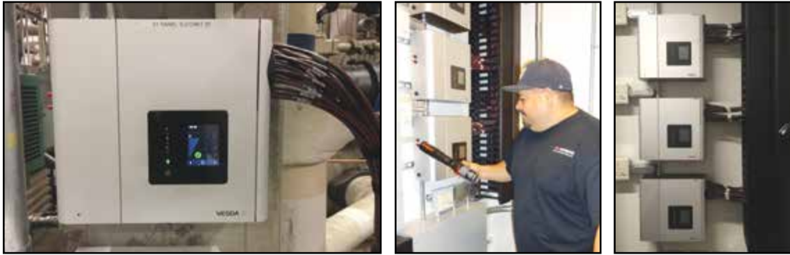
Smoke detection equipment must distinguish smoke from a fire vs. ride effects and dust. A centralized detector allows for annual testing in an accessible location. COURTESY XTRALIS
