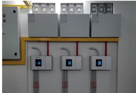
HFT is a flame-retardant halogen-free polymer conduit introduced to the safety industry, which are designed to offer fire-retardant properties without degrading their functional performance including impact resistance. Most importantly, its characteristics of being able to bend easy within the extrusion and high temperature rating.
