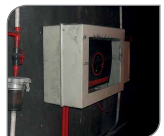
Figure 2 - VESDA VLI in protective enclosure
