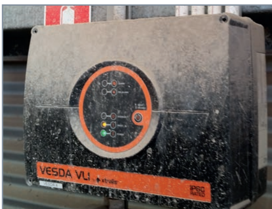
Figure 1: VESDA VLI detector in dirty environment without protection
