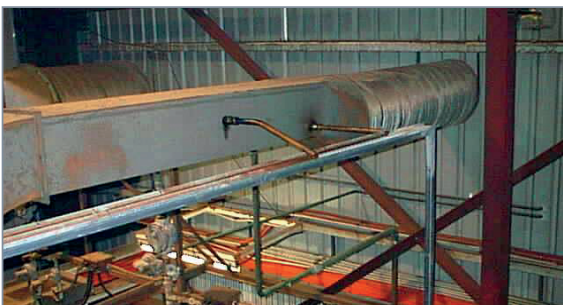
Figure 1 - Roaster Oven Exhaust Sampling
