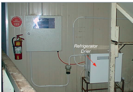
Figure 4 - ASD with refrigerator drier
