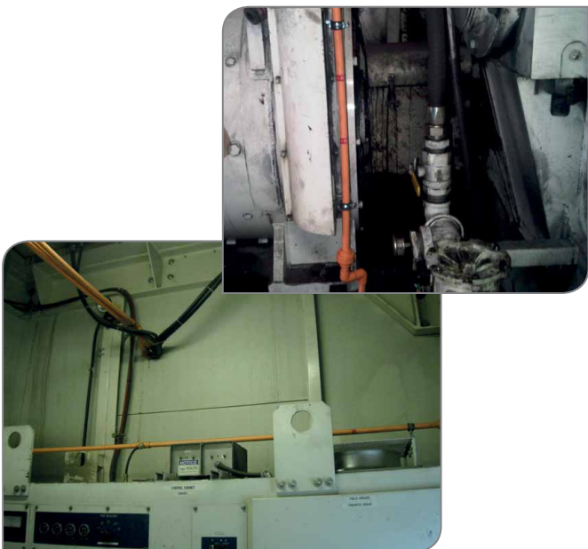
Figure 5 - Sample pipe in Shovel
