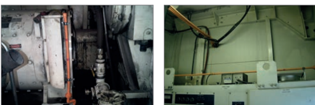
Figure 5 – Sample pipe in Shovel
