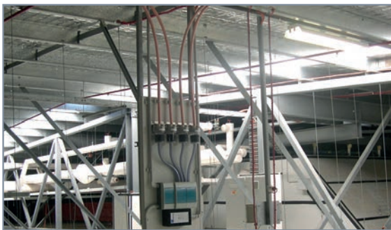
Figure 4 – Detector and Pipes in Roof Space
