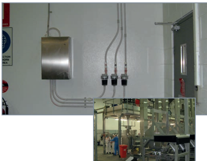
Figure 4: VESDA System in Food Production Facility
