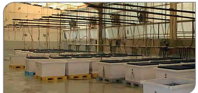
Figure 2 - Battery Filling / Charging Room
