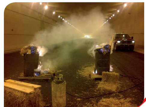
Tunnel smoke testing
