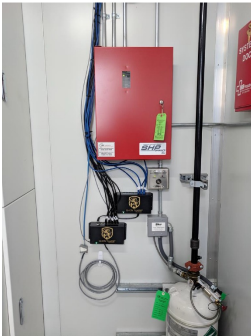
Figure 9: Controllers Mounted Below Fire Control Panel
