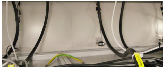
Figure 2: Monitoring Sensor Placement Above Racks - Mounted to Walls
