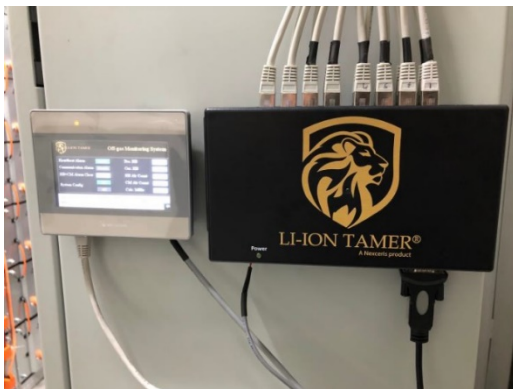
Figure 11: Controller Connected to Monitoring Display
