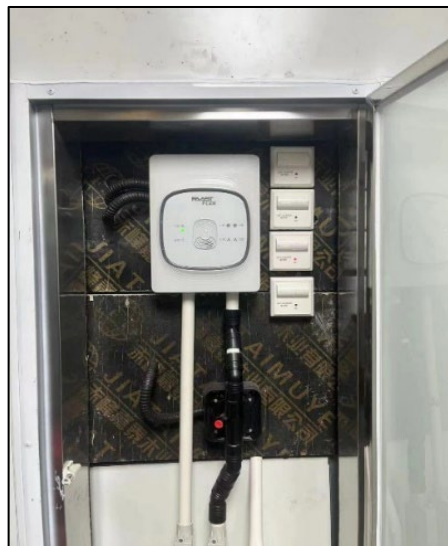
Figure 2: FAAST FLEX & VESDA XCL Mounting
