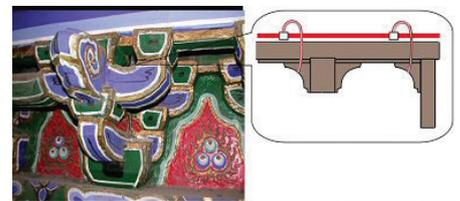
Tiny capillary tubes can be dropped from the pipes and hidden within the decorative detailing. The tubes can even be painted to be completely camouflaged.
