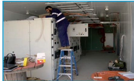
Capillary tubes branch off the main VESDA sampling pipe and into the equipment cabinet, allowing the earliest possible warning of smoke within the cabinet.
