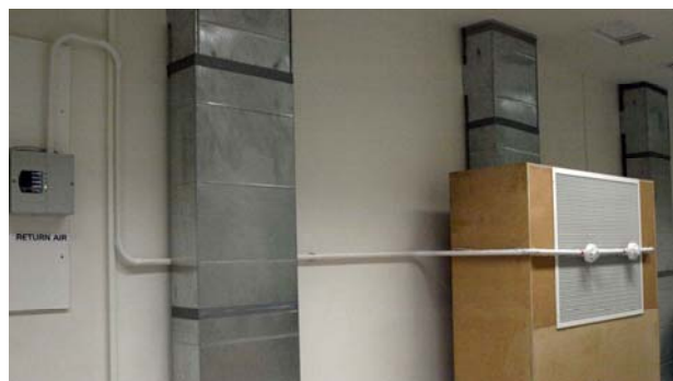
Figure 6 – VESDA System Layout – Return Air Protection.
