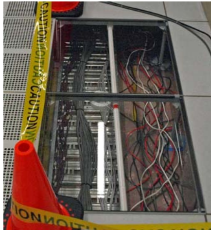
Figure 9 – VESDA in Floor Void Protection (illustration).
