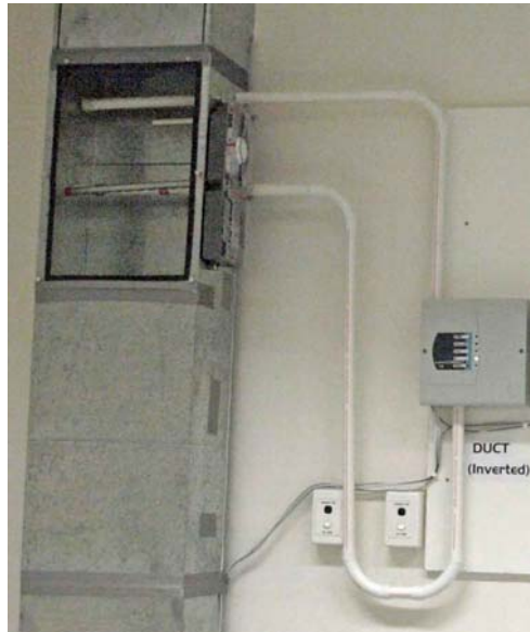
Figure 7 – VESDA System Layout – Duct Protection.
