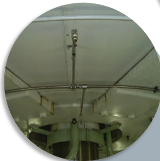
Sampling pipes installed on a HYDRO generator sample near the likely risk.
