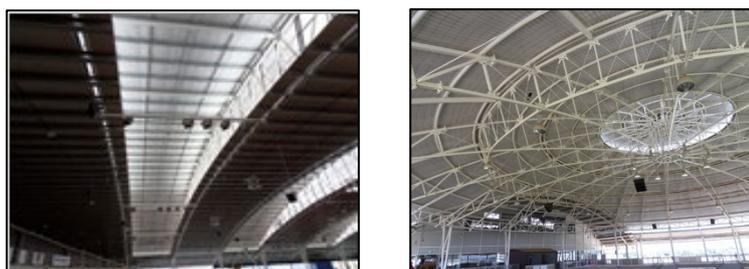
In order to meet the natural smoke ventilation requirements of the Fire Safety Engineering Report, the centre design is permanently open to natural atmospheric conditions. Metal louvers were part of the solid window sections on the first floor level, opened and closed according to the conditions. The open stock entrances to the Sales Ring / Warm Up Arenas, all influenced the original detection performance.
