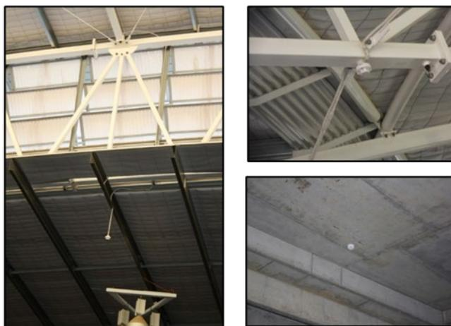
In view of the number of nuisance alarms from the ionizations detection system, AELEC management sought an independent appraisal of the system from consultants (Fire and Safety Technologies Pty. Ltd.). This company was ultimately engaged to survey the installed system and report on the findings. The findings covered various aspects of the designed system and clearly made reference to the fire detection system.
