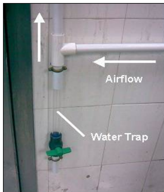
Figure 2: Water Trap Arrangement
