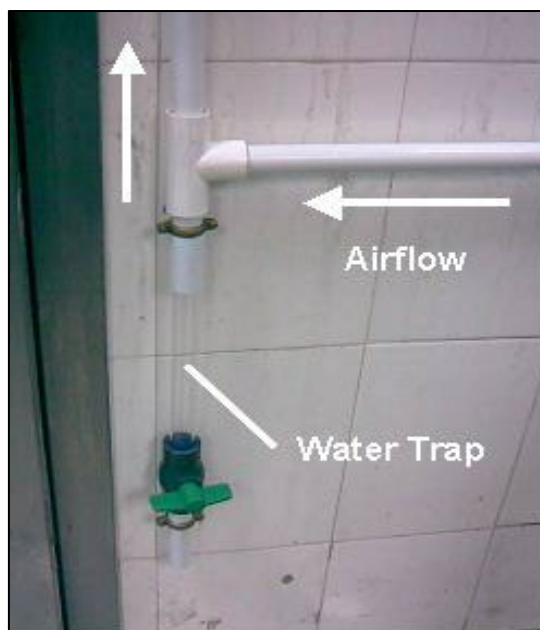
Figure 2: Water Trap Arrangement
