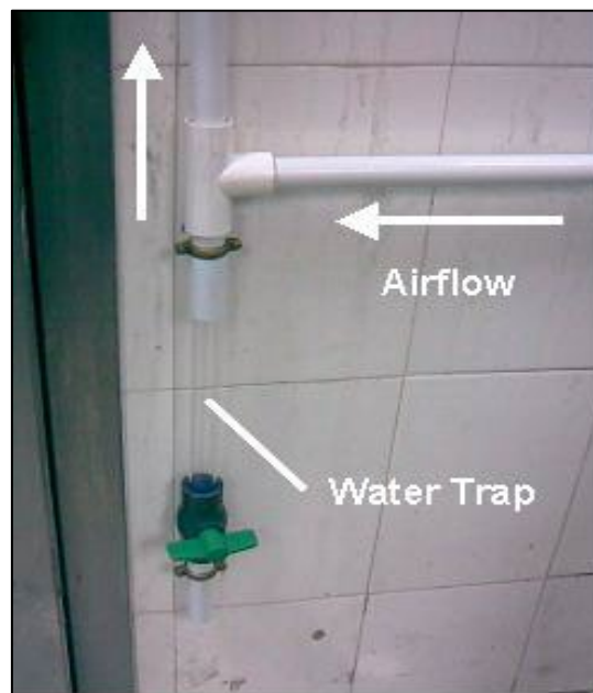
Figure 2: Water Trap Arrangement
