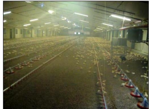
The example below is from a site where water mist is sprayed every few minutes, 24/7 to maintain a humid environment. In a trial using OSID (Imager 10°) over a distance of ca. 40-50m, no water droplets or condensation occurred on the Imager or Emitter lenses. The graph below shows a 30 min period. There is little differentiation between UV and IR, hence the site operated without false alarm or faults.
