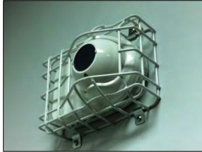
OSID detection is very convenient for detection in sports arenas, etc. To protect Imagers and Emitters from vandalism and accidental damage a steel cage, OSID-WG, should be used.
