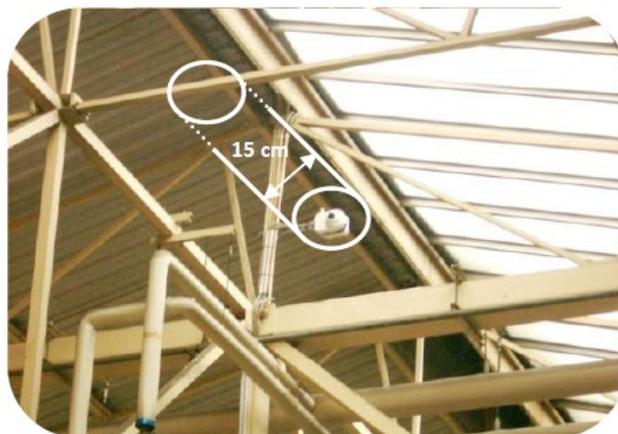
Hence the OSI Imager requires a free transmission space path of 15 cm/5.85" diameter 'minimum' at all times. Use 20 cm/7.8" minimum rather than 15 cm/5.85" if multiple openings are lined up like i.e. openings in consecutive smoke curtains.
