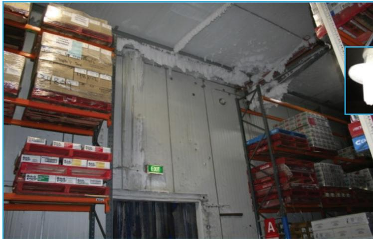
smoke. In some instances the only solution is to remove the iced up section of the ASD pipe network and fit a new pipe.
